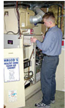
Todd Martin, lead home energy auditor, testing airflow using a balometer.
