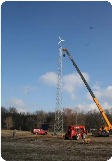
Halco crews install Guilford and Beth Mack's wind turbine in the field by their house.
