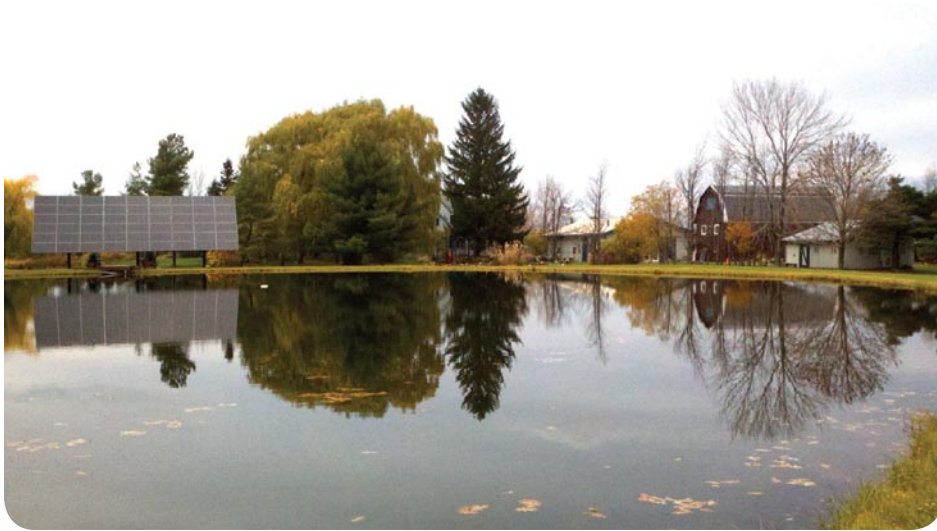
Noble House Farm Bed & Breakfast pond with solar panel on its shore.
