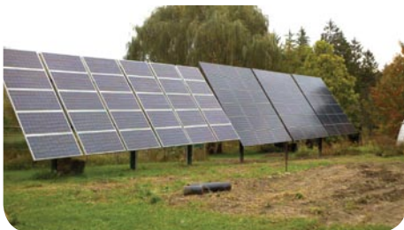
The new and existing solar panels side-by-side.
