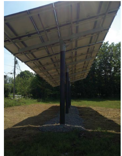
The solar panel tilt can be adjusted seasonally to follow the sun’s angle in the sky.
