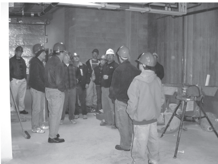
The tour began in the basement where Halco foreman Leo Fenner (white hat) explained the HVAC system.
