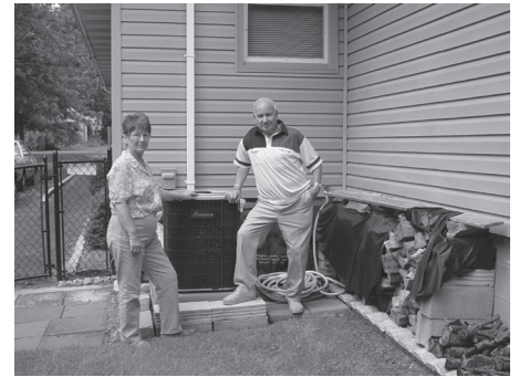
Maddalena and Matthew beside the Amana condensing unit in a corner of their back yard.
