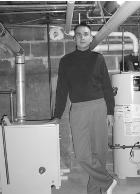
Scott Ritchie stands between his new boiler and water heater.
